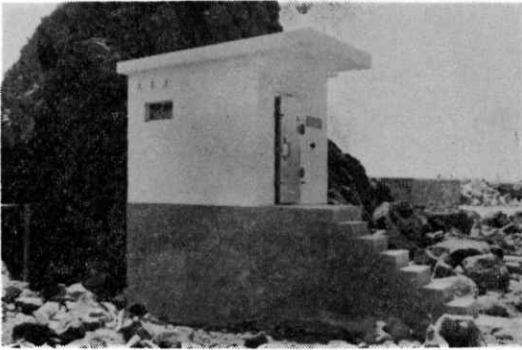
驗潮所外觀 Appearance of the tide-gauge station.
