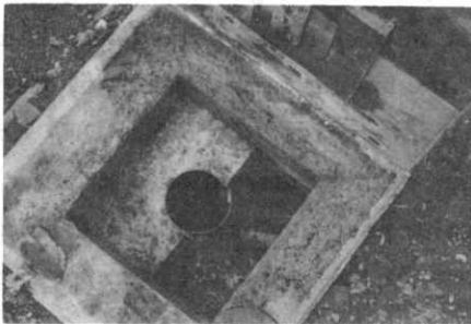
写真-1 観測井地表孔 Exit of cable.
