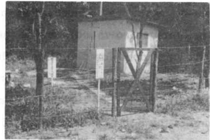
写真-3 観測井測定室 Measuring lodge.
