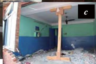
Fig. 3.14 At Gongabu, RC frame buildings were tilted (a,b). A shear crack in the first floor (c) (Photo. by T. Ohsumi).
