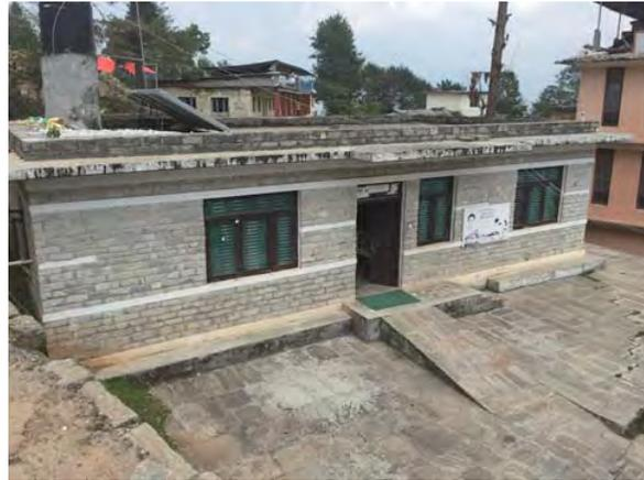
Fig. 5.3 Seismic RC band for stone and brick masonry (NSET promoted in Dolakha, Nepal) (Photo. by H. Imai) (upper figure from Arya (2013)<sup>4</sup>).
