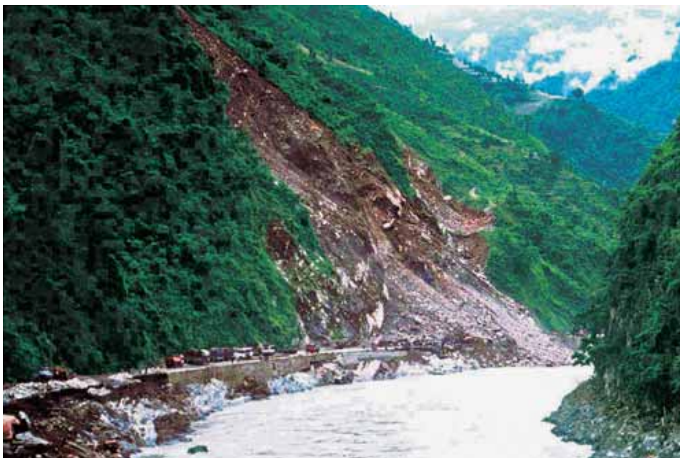
Fig. 3.6 An over view of Jogimara landslide which damaged the Prithivi Highway (Muglin to Kathmandu road) in the Middle Mountain of Nepal. This photo was taken just after disaster in July 1993.
